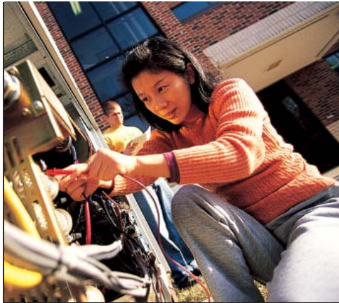
Above: Mechanical Engineering graduate student Xiahong Liao troubleshoots the microturbine at the Cooling, Heating, and Power (CHP) Integration Test Center at the University of Maryland. The goal of the center is to deliver a small packaged CHP system that is grid independent.
