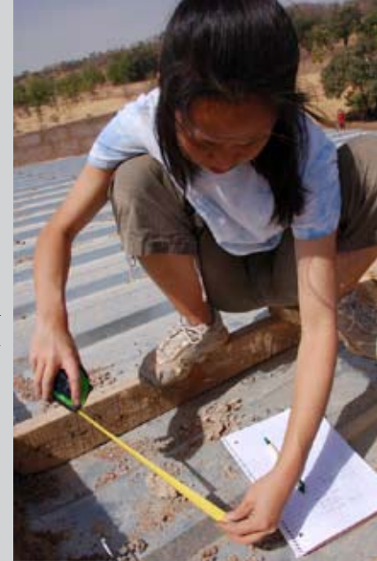
KANA MATSUI INSTALLS A SOLAR PANEL ARRAY
