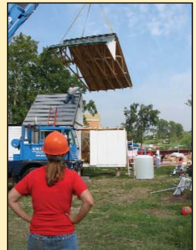
Right: Putting it together just to take it apart — a crane lifts a roof section off the house and onto a flatbed truck to be taken to the National Mall, while teammate Robyn Hladish looks on.
