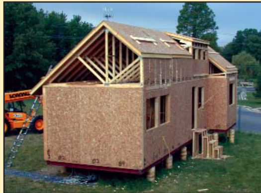
Above: The shell as it looked in June. The walls were pre-fabricated modular sections that fit together like a giant jigsaw puzzle. While the insulating properties of this type of building are much higher than regular stick-built homes, modular building also made building and transporting the house easier.
