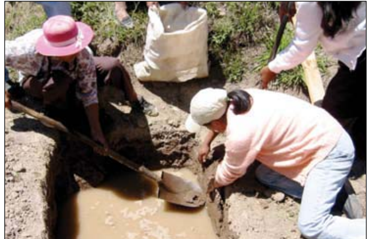
Above: Villagers dig a well in Raric that allows the testing of water quality with a perc test, which will help the EWB-UMD team evaluate the potential potable water resources in the area. The water was tested for Ph, iron, alkalinity, hardness, chlorine, nitrite and nitrate levels.
