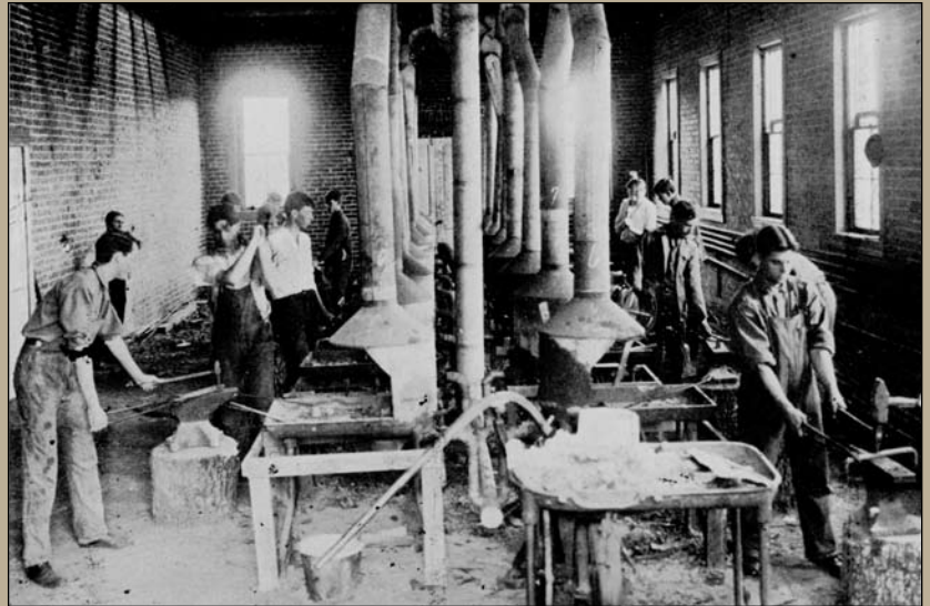
Fabrication Shop - photo marked 'Mechanical Engineering', date and photographer unknown. University of Maryland Archives.
